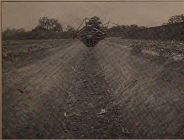
Wheel Ditcher operating under Gasoline Power. Figure 64.
